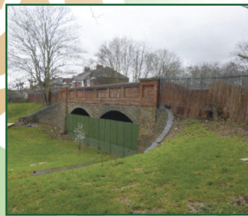
The original bridge under Belmont Road leading to what are now the grounds of Park View School
