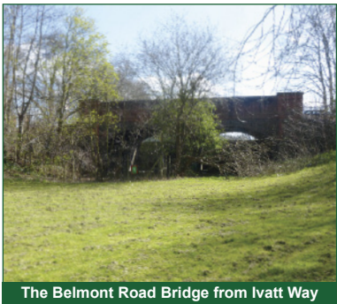
The Belmont Road Bridge from Ivatt Way
